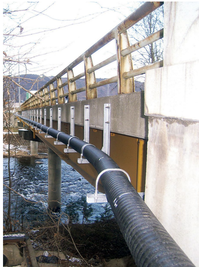
橋梁地覆横曲げ配管
