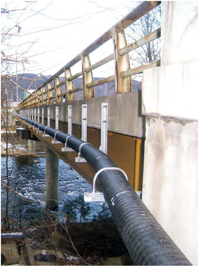
橋梁地覆横曲げ配管
