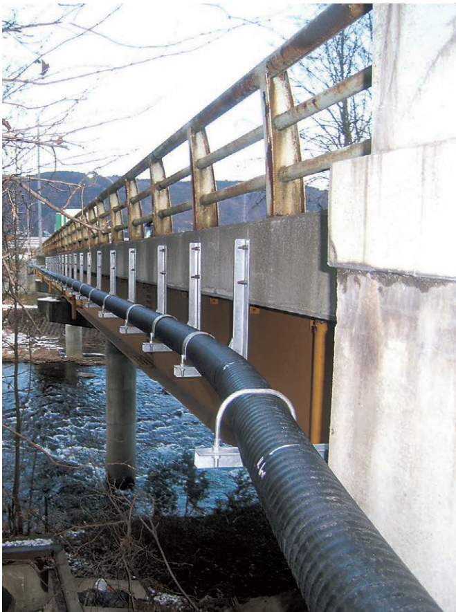
橋梁地覆横曲げ配管
